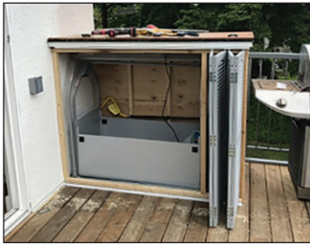
Unique outside deck installation
